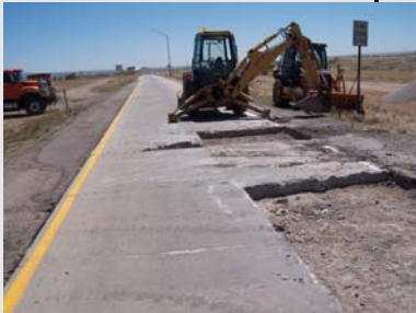
POE Eastbound On Ramp
