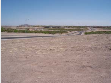
Las Cruces State Police District Office Construction Site
