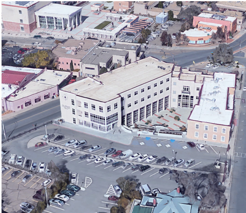
View to the North
