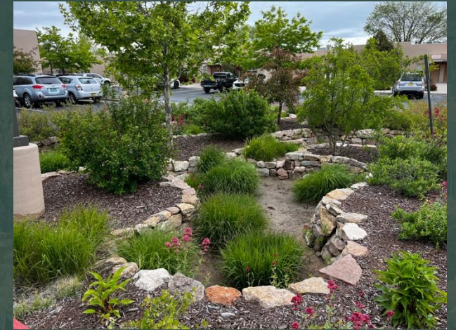
Green stormwater infrastructure
