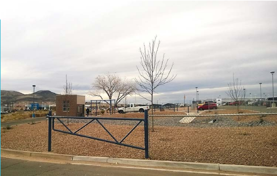
Vehicle Gate and Guard Shack
