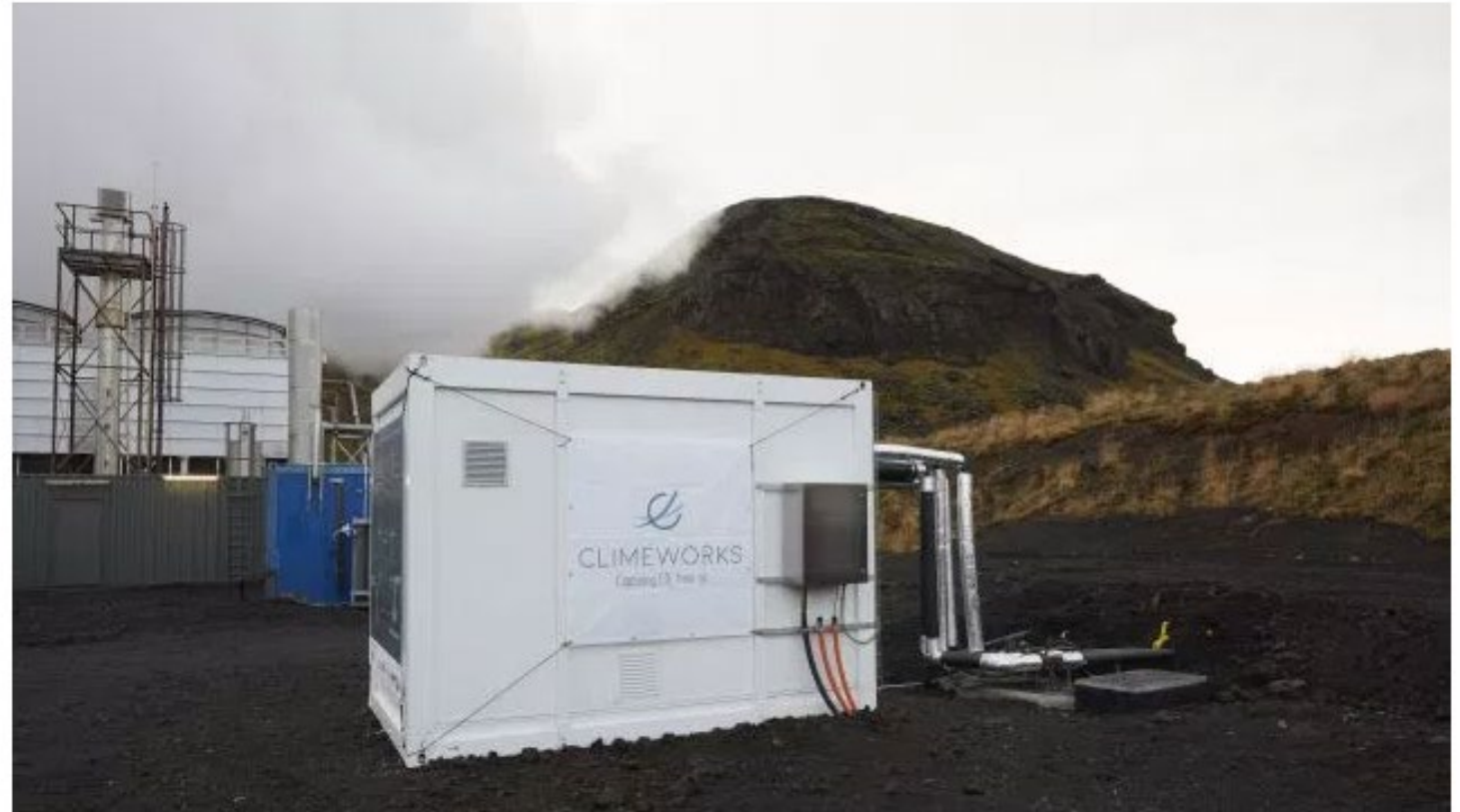
📷 Direct air capture unit along with the cooling towers of the geothermal power plant in Hellisheidi, Iceland. (Climeworks/Zev Starr-Tambor)
