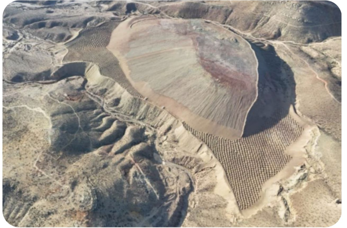
Smoothing out this former rock quarry in Dona Ana County earned the Las Cruces District Office of the U.S. Bureau of Land Management a 2025 Excellence in Reclamation Award.
