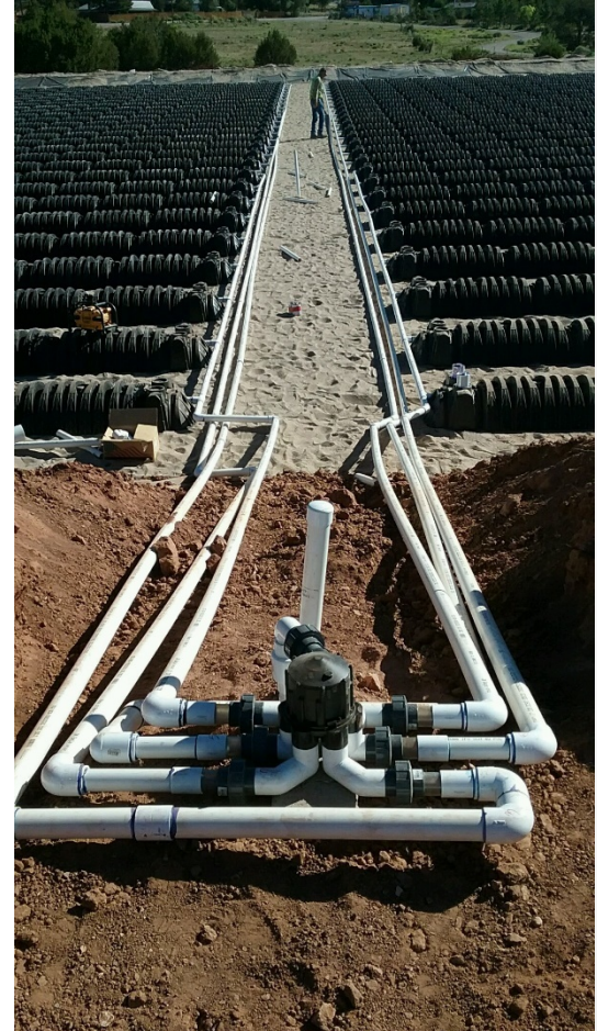
Bluewater Lake State Park Evapotranspiration System
