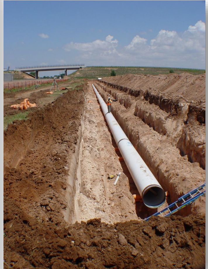
FW2 Pipeline Construction
