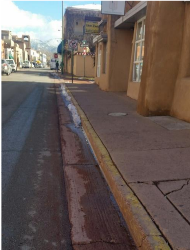
Figure 41: Downtown Santa Fe – Curb Providing Opportunity for Microtrench Construction
