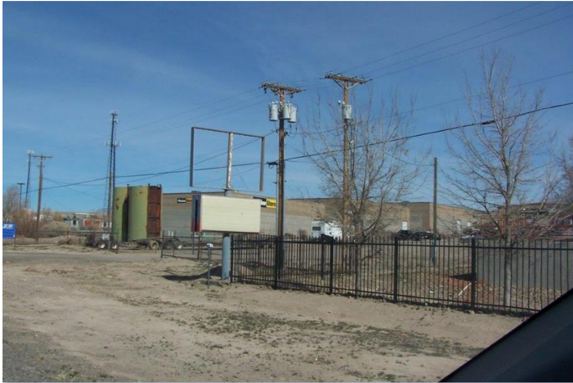
Figure 37: Telephone Lines on Broadway Boulevard
