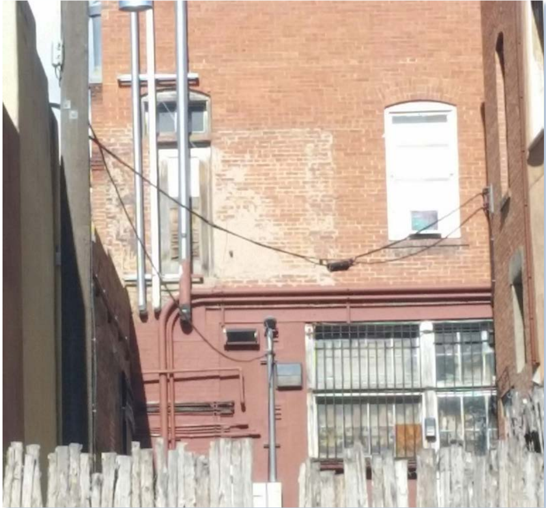
Figure 40: Downtown Santa Fe – Ad Hoc Telecommunications Cabling Hanging from Building to Building
