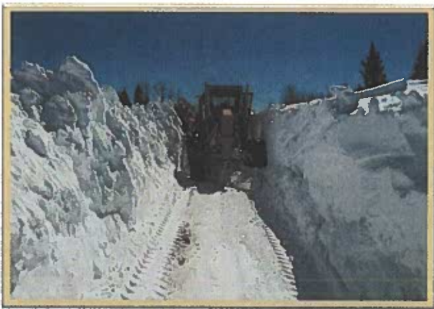
US 64 Opening Roadway between Tierra Amarilla & Tres Piedras
