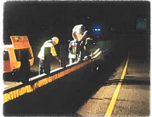
Glare Shield Repair, I-25
