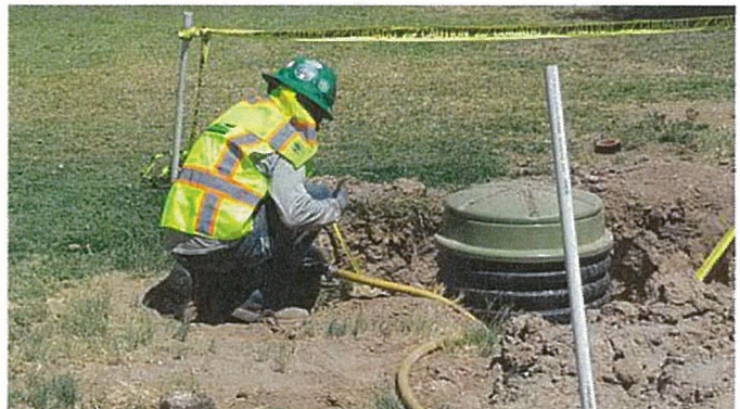
Grinder Pump Installation
