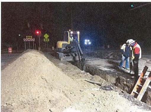
Installation of 6" Sewer Lines along Molina Drive
