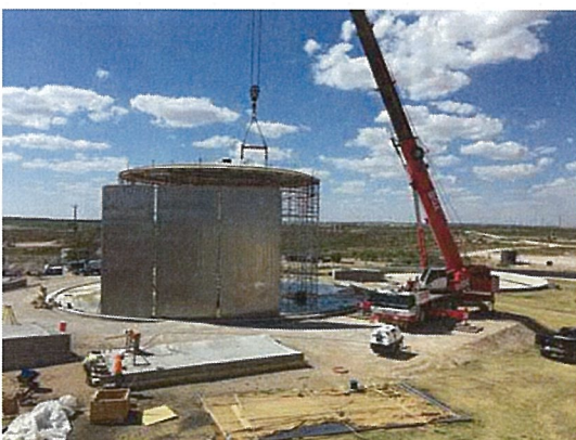
Placement of Tank Panels
