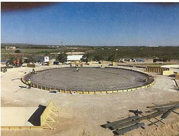
Concrete Form and Rebar Tank Foundation
