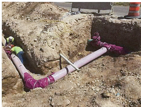
12 Inch Reuse Pipe Installation
