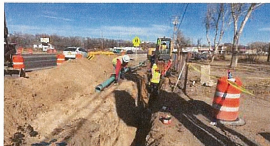
Peralta Installation of 8" Sewer Line along HWY 47
