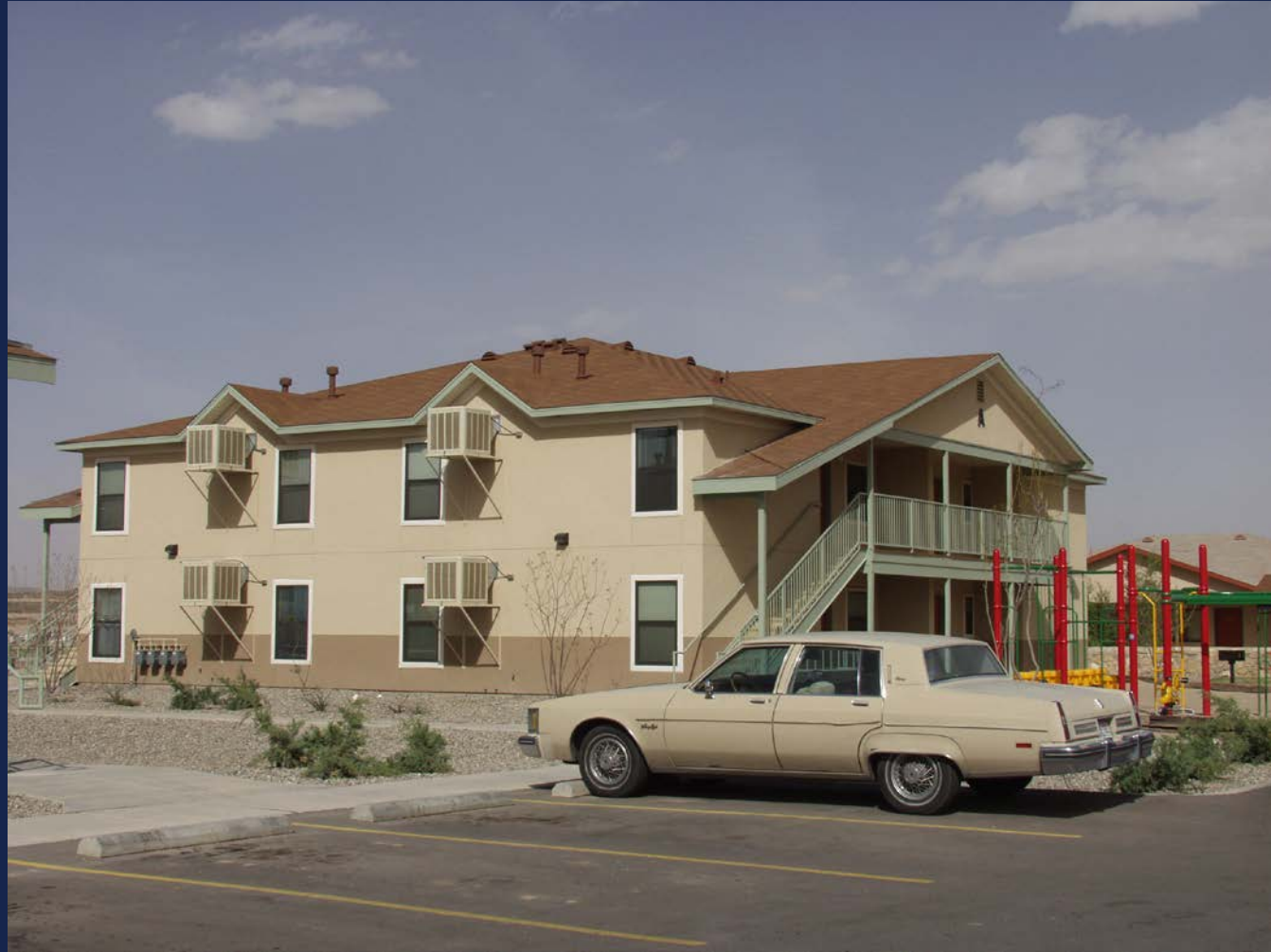
Franklin Vista Apartment Complex Anthony, NM
