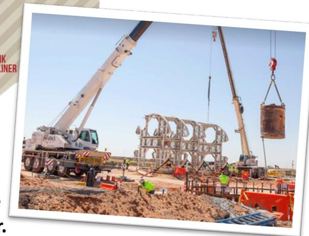
A bucketload of excavated material is lifted from the utility shaft. The Galloway work platform is at center.
