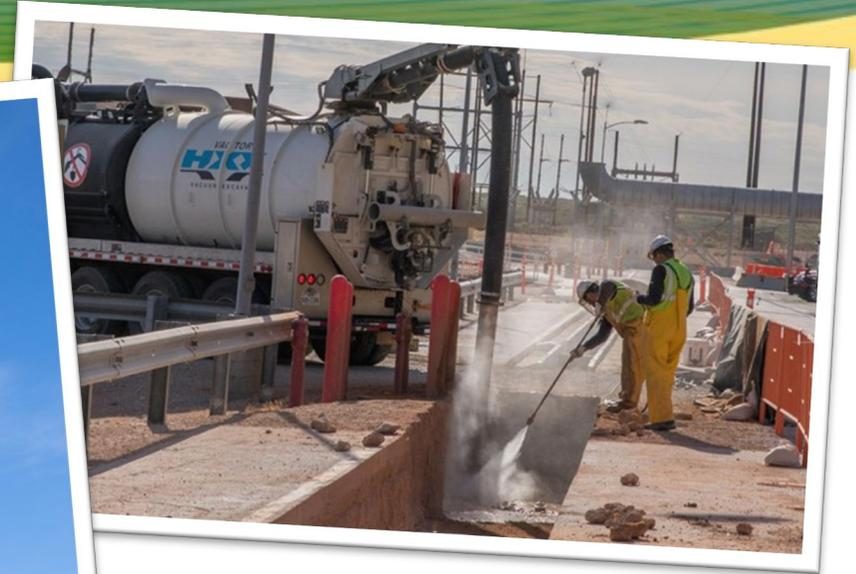
Multiple hydro-excavations are happening at WIPP for new air, fire water and fiber optic lines.
