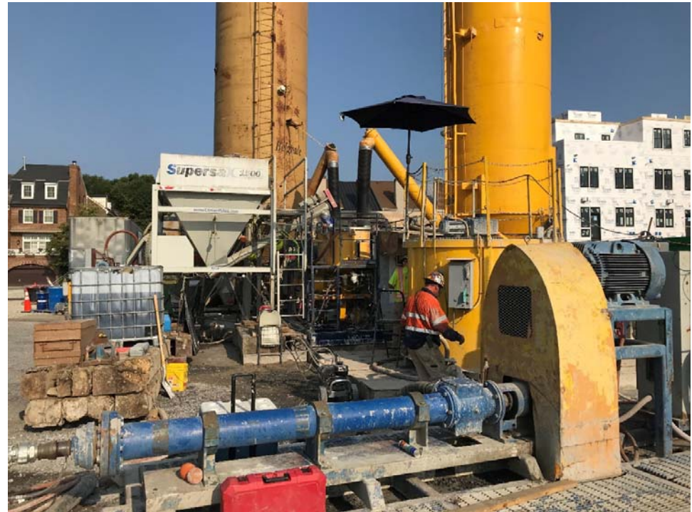
Pressure Grouting Equipment
