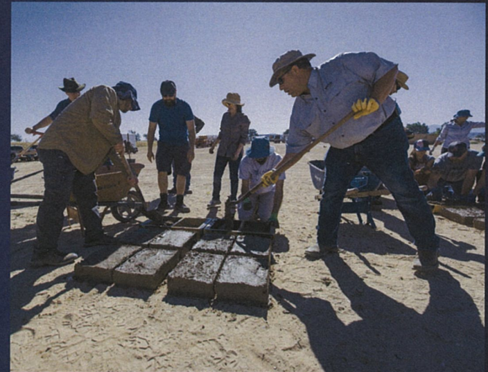
Lab volunteers work on an adobe brick-making project to support a housing renovation at a neighboring Pueblo.
