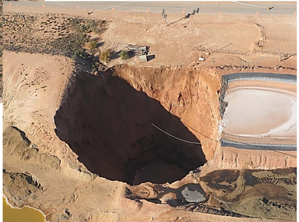
Loco Hills Disposal – November 2008
