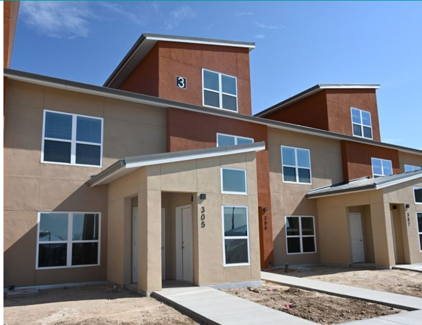
East Paraje Apartments, a 20-unit development in Laguna Pueblo. Housing New Mexico provided $7.8 million in financing to the project.
