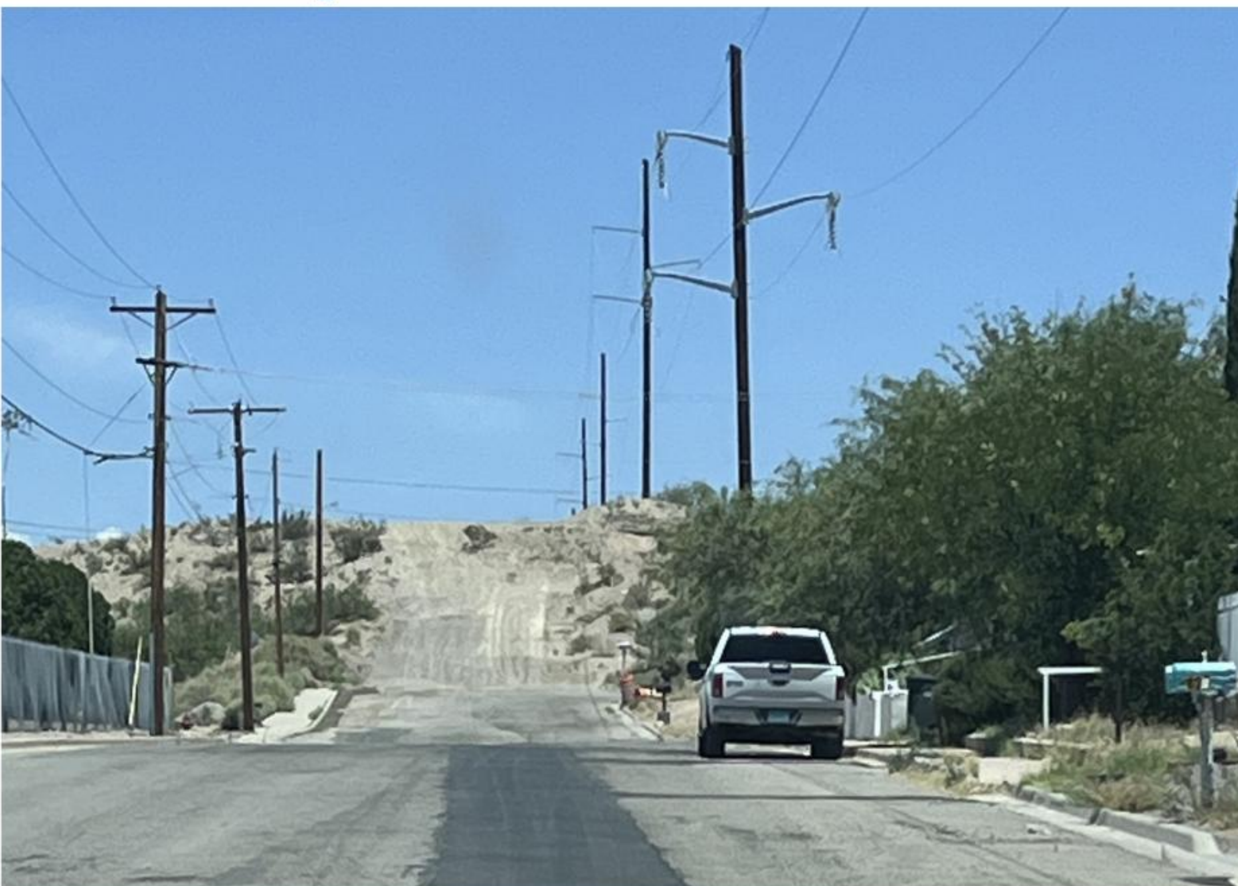
Trench patch, City street — new line abandoned old pavement on either side
