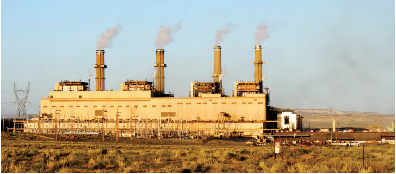
Two of the four units at the San Juan Generating Station, located near Farmington, New Mexico, are slated to be closed in 2017. PNM has discussed closing the remaining two units in 2022. As coal plants retire, utilities are deciding which energy investments to make to replace them.
