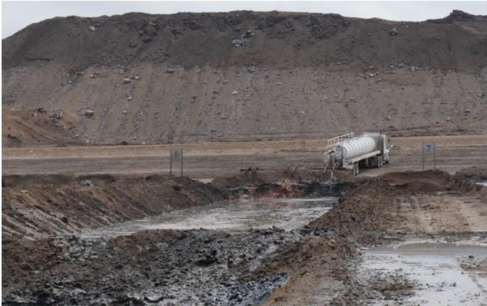
Oil and gas wastewater is dumped from a truck into one of a series of unlined pits at the R360 waste disposal facility outside Hobbs, New Mexico, 2019. Photo credit: Melissa A. Troutman.
