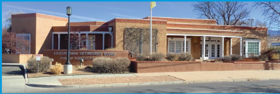
ERB Building purchase
