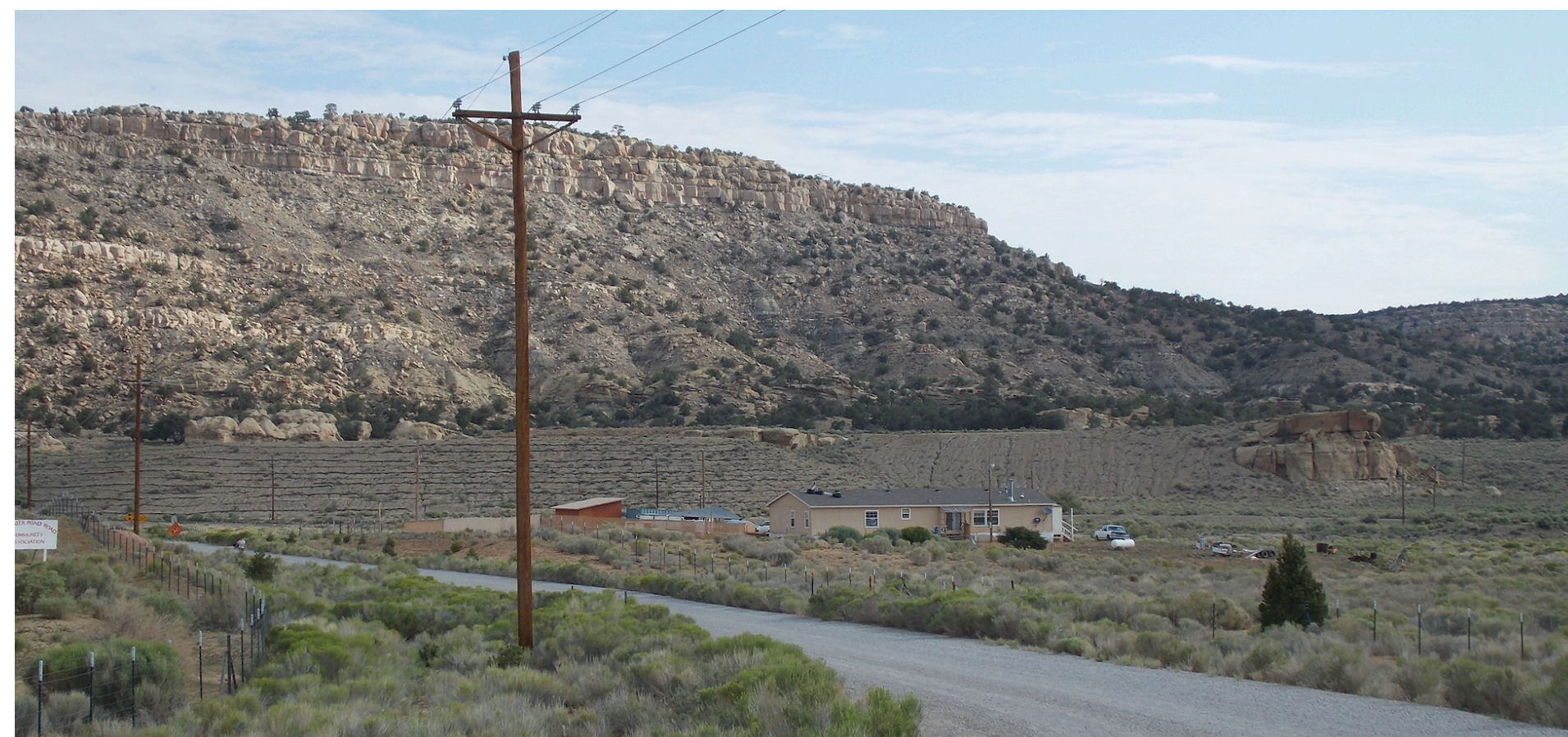
Northeast Church Rock Uranium Mine Waste Pile in Red Water Pond Road Community on Navajo Nation
