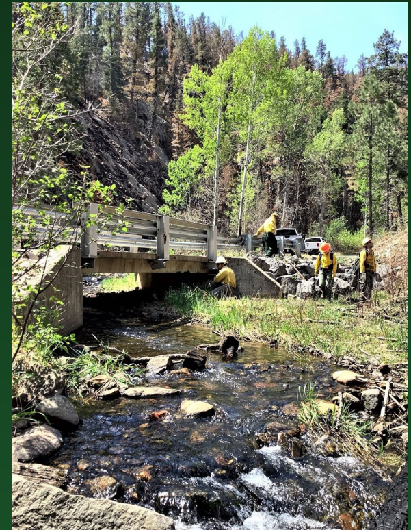
BAER Specialists assessing Culvert off of Forest Service NFSR 156 Road in Hermits Peak/Calf Canyon Burned Area.
