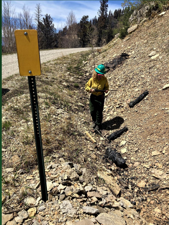
BAER Civil Engineer Lisa Archuleta assessing road culverts for drainage.
