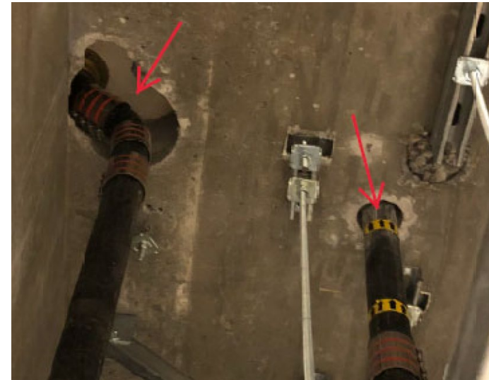
Fire Barrier Deficiencies in RLUOB
