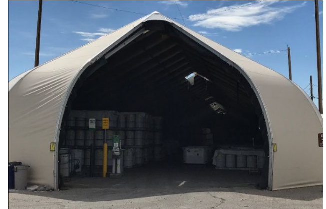
Dome 49 at LANL's Area G
