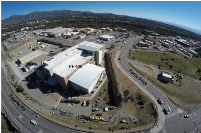
Aerial View of RLUOB/PF-400
