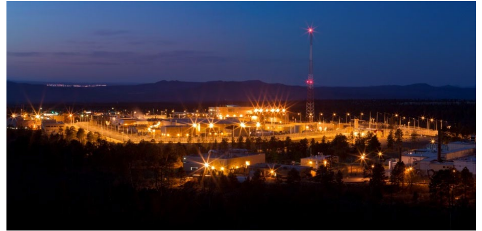
LANL Plutonium Facility
