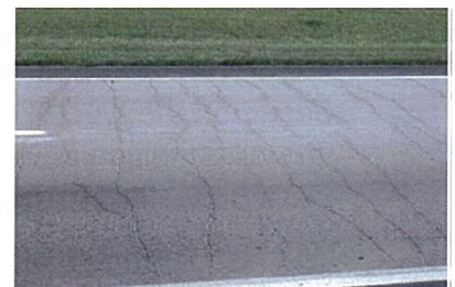
Transverse Cracks
