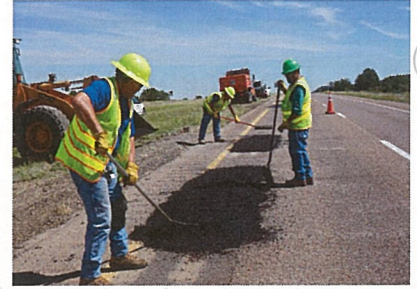
pothole patching
