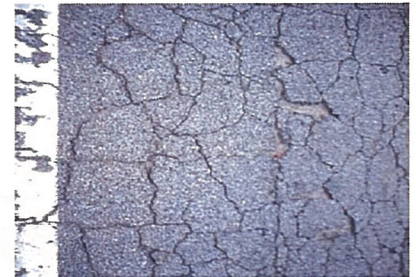
Alligator Cracking
