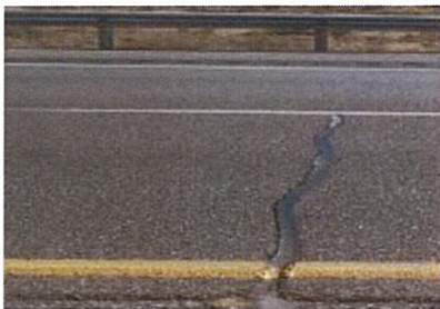
Transverse Cracking
