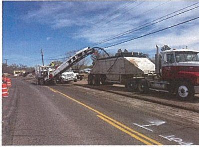
cold milling asphalt pavement
