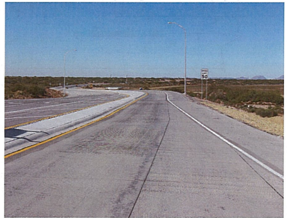
Rigid (Concrete) Pavement
