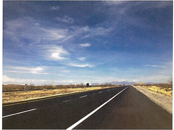
flexible (asphalt) pavement
