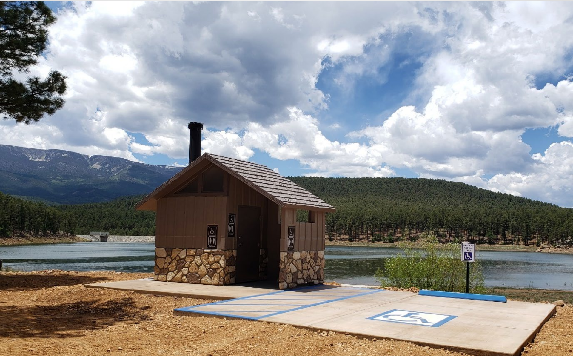
Park Renovation Morphy Lake State Park, Mora County - $800,000
