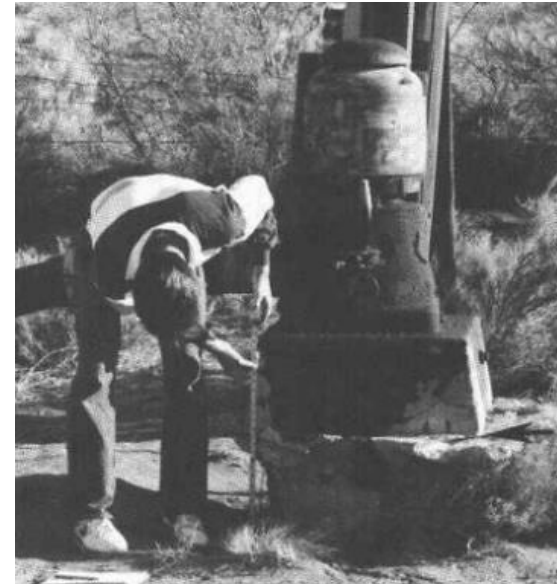
Land subsidence of over 1 ft (1988)
