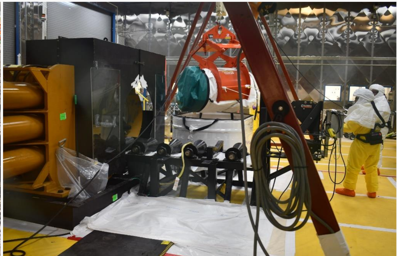
CMP segment lowered into a standard waste box
