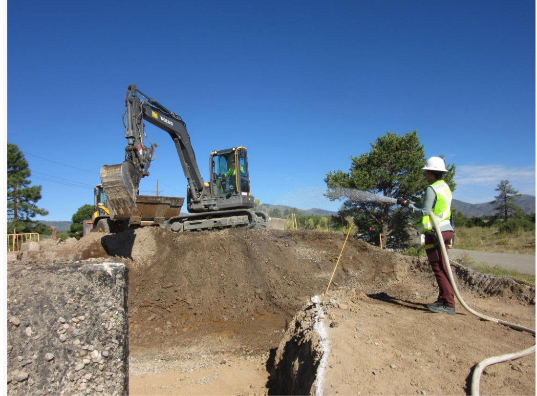
Excavation of contaminated soil from LANL legacy operations
