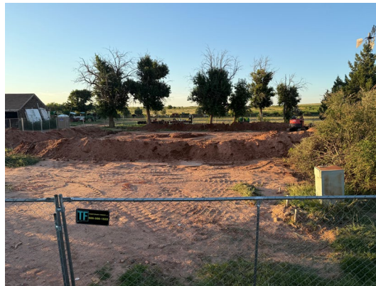
Current Construction Site
