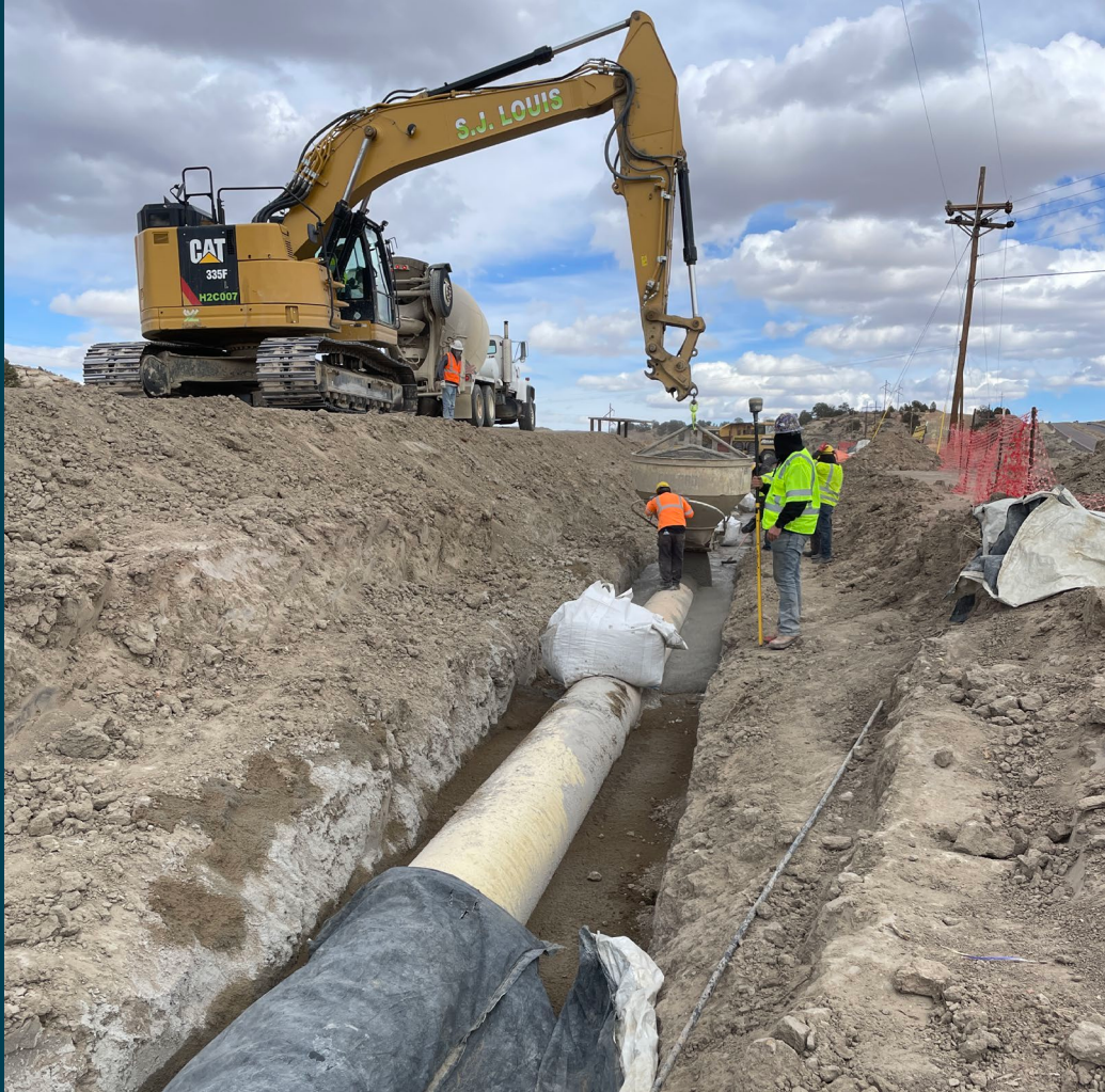
Navajo Code Talkers Pipeline Completed May 2025
