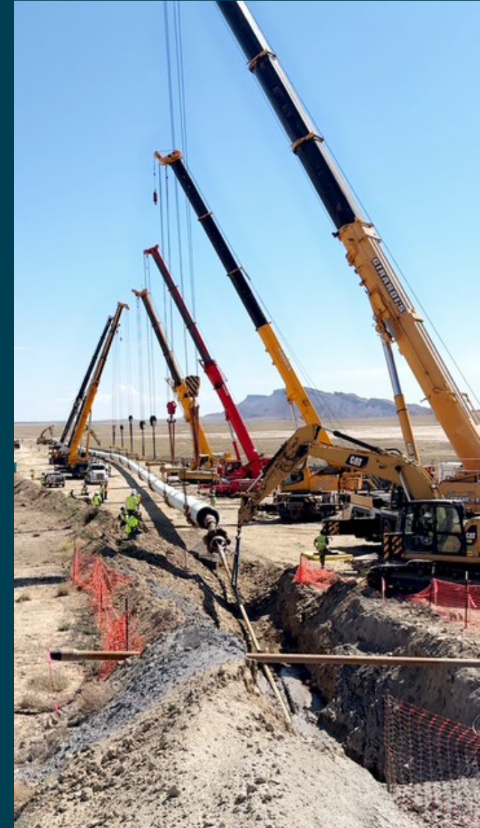
Reach 4B HDD Pullback – June 2025
