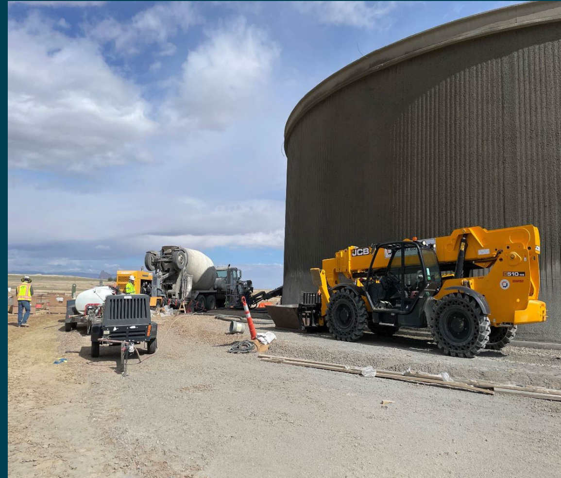
Pumping Plant 2 Storage Tank Construction – June 2025
