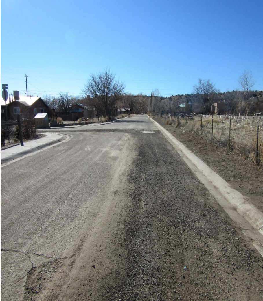
Santa Clara Sewer Line Project
