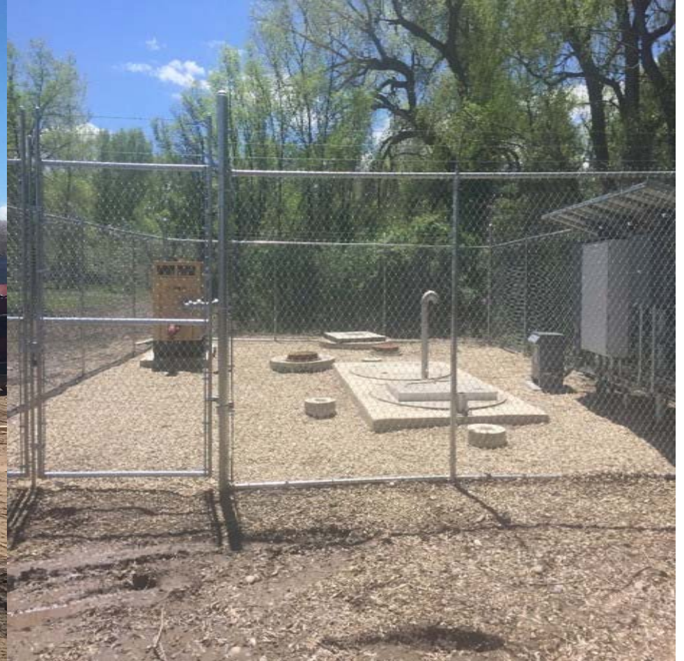
Taos Pueblo Water & Sewer Expansion
