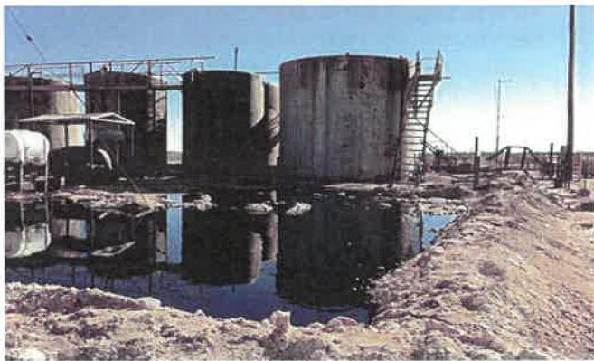
Photo of an unlined wastewater pit.
