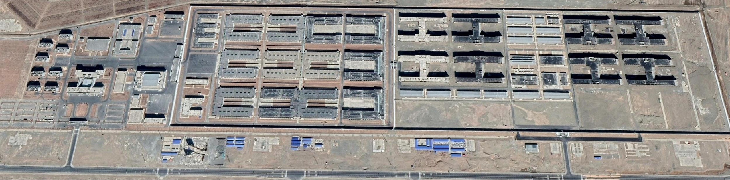
A close-up look at the construction
