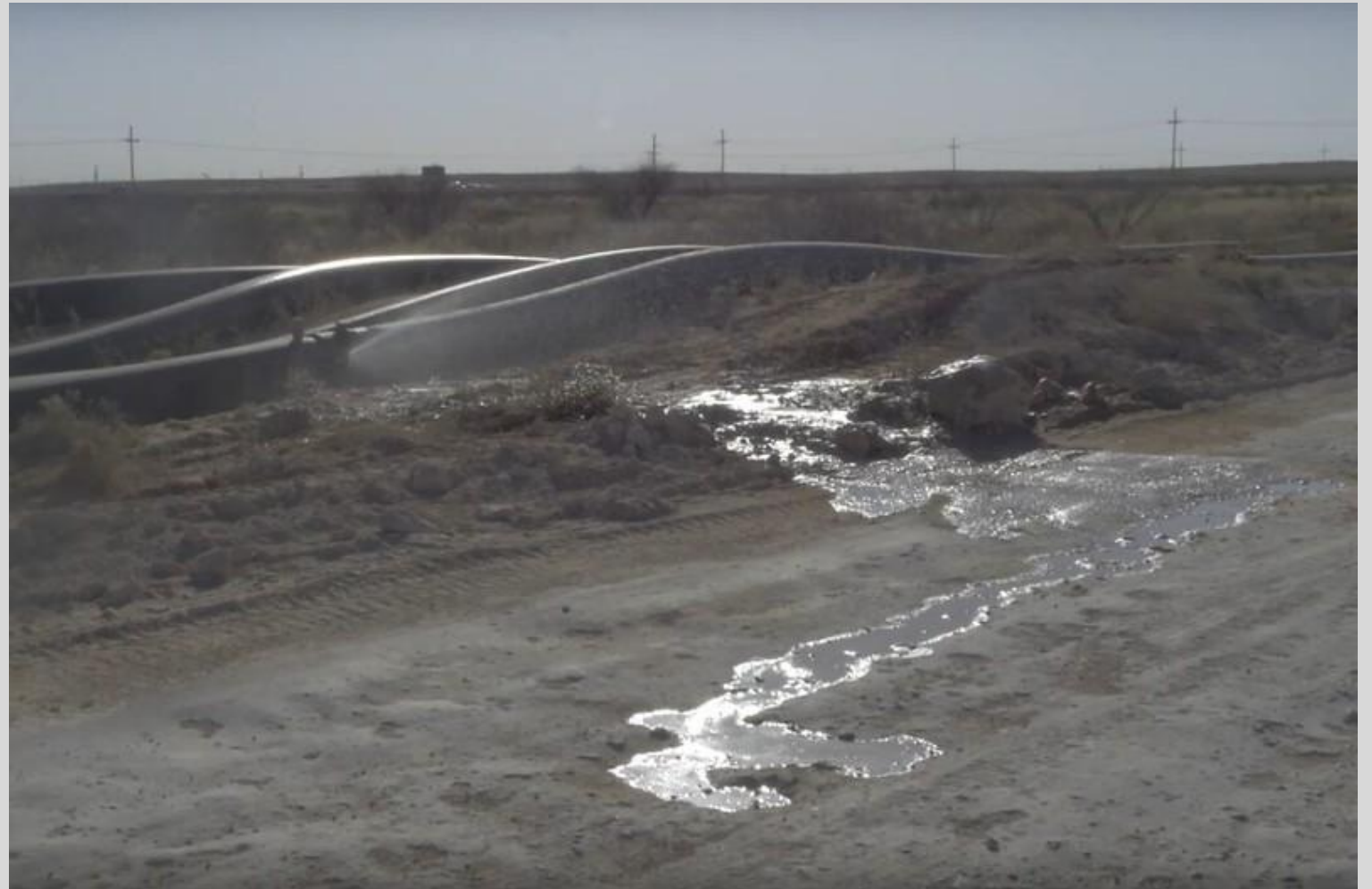
Photo by Melissa A. Troutman: An active spill of smelly, discolored liquid from a produced water pipe snaking across Eddy County in February 2023.
