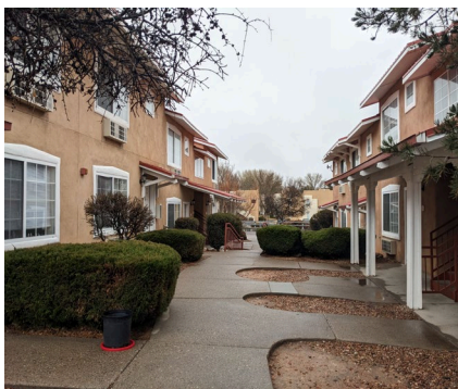
Figure 8. Santa Fe Suites encompasses 123 supportive housing units for chronically homeless and low-income individuals
