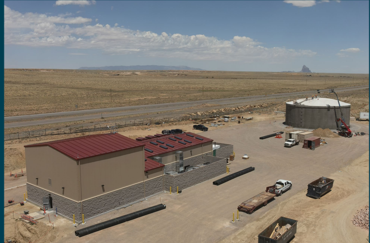
Pumping Plant 3 Aerial Photo (looking NW towards Shiprock) – June 2025
