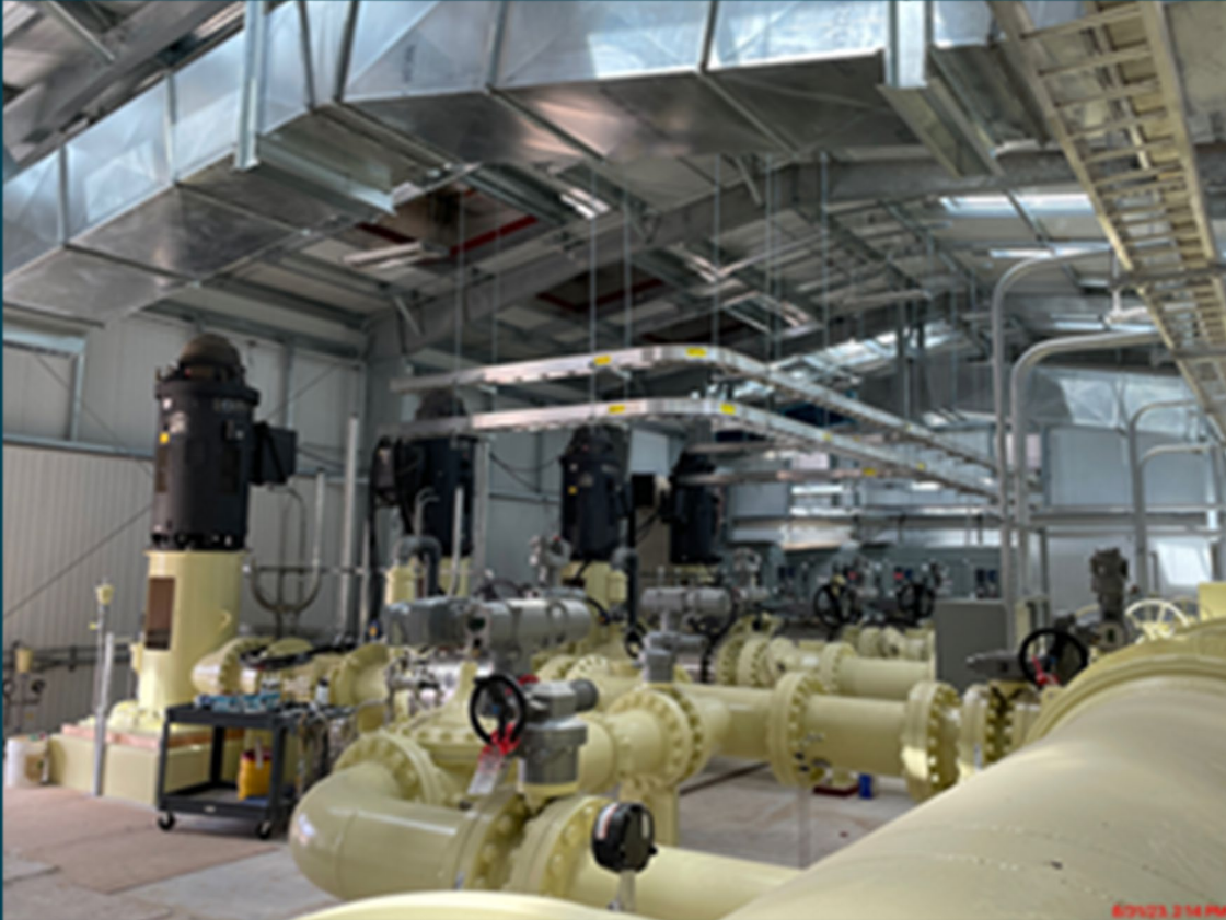
Pumping Plant 4 Interior Pump Room – Completed in April 2025
