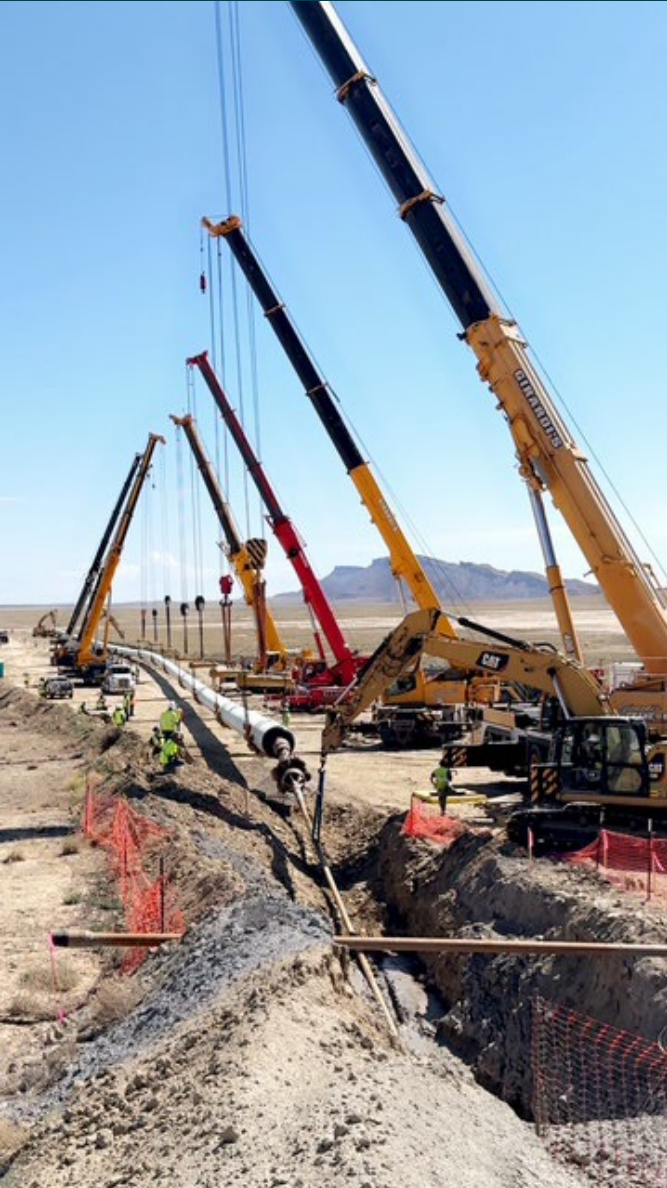
Reach 4B HDD Pullback – June 2025
