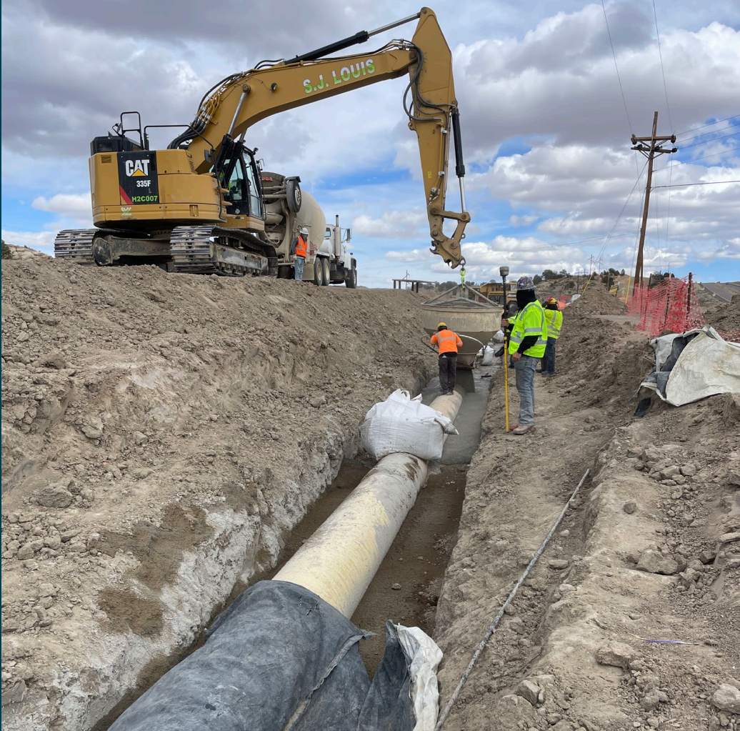
Navajo Code Talkers Pipeline 9 Completed May 2025
