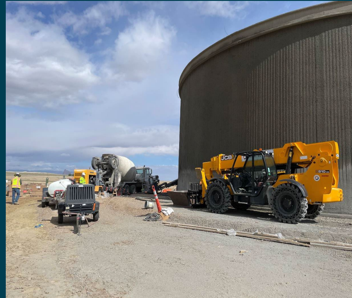
Pumping Plant 2 Storage Tank Construction – June 2025
