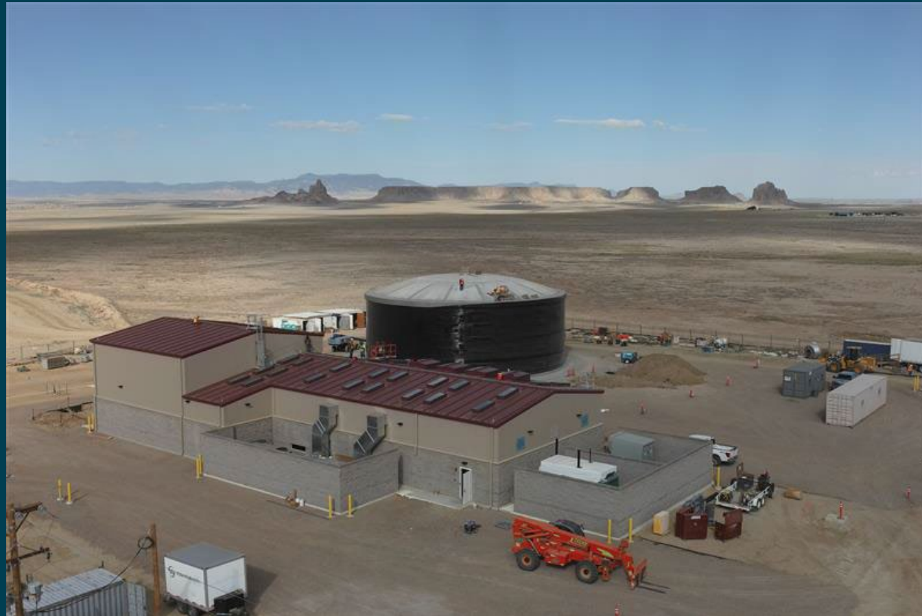
Pumping Plant 2 (looking west towards Table Mesa) – June 2025
