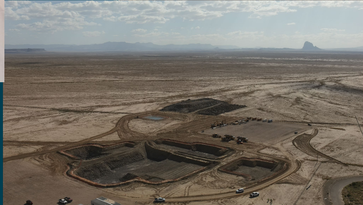
Aerial Photo of SJLWTP Construction – 6/23/2025
