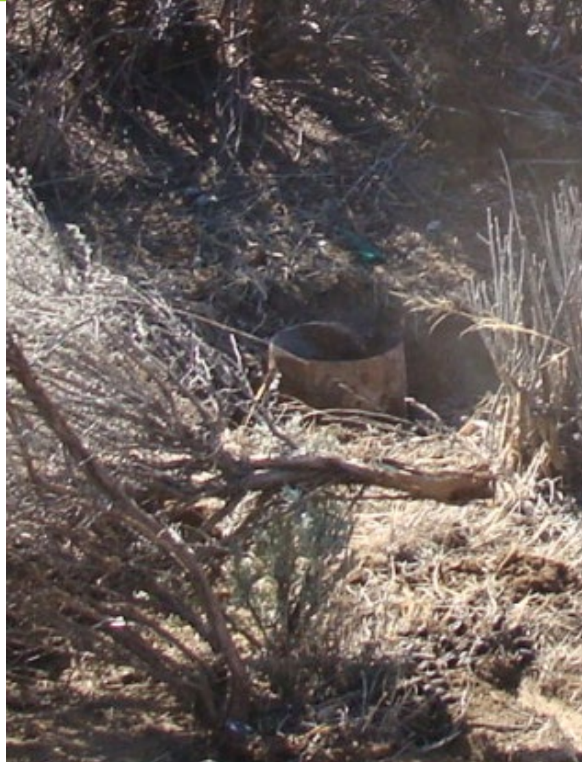
Abandoned Well previously buried underground
