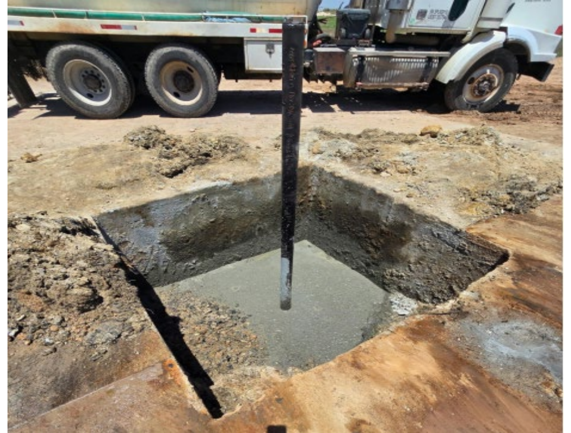
Post plugging, dry hole marker set
