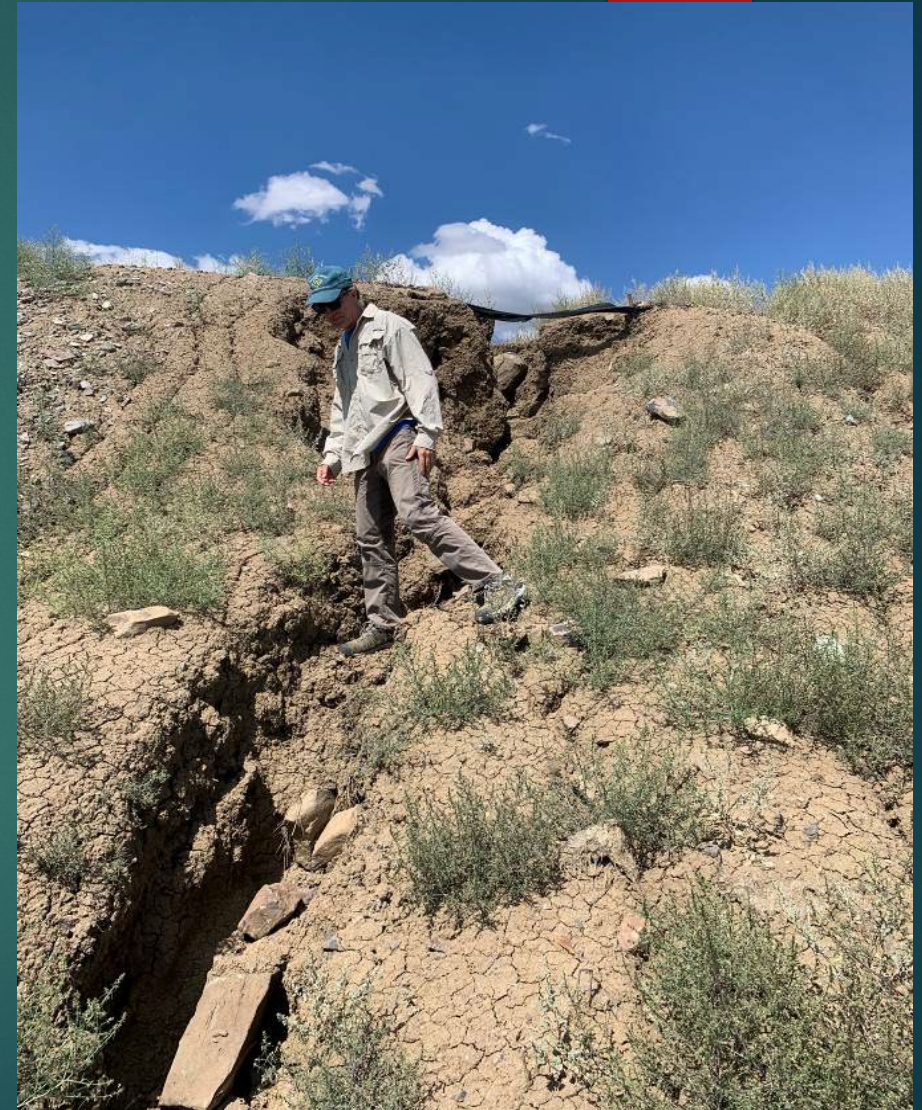
Erosion at J.J. No. 1 Mine
