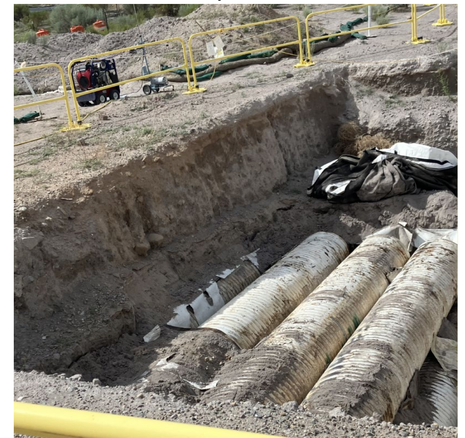
Excavation of Corrugated Metal Pipes at Area G. 10
