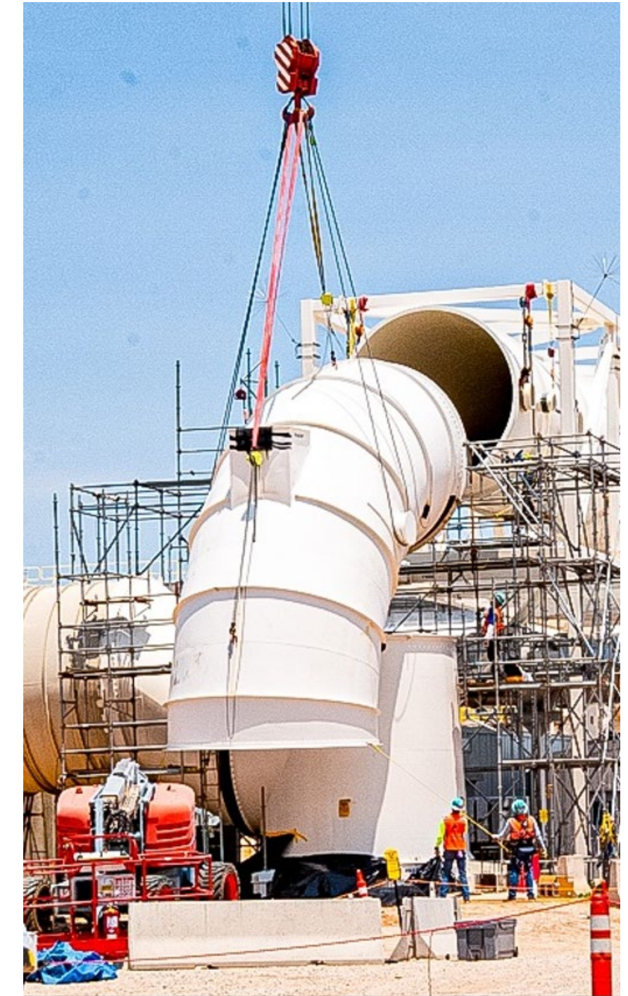
Final connection in late 2024 followed by startup of UVS in June 2025.
