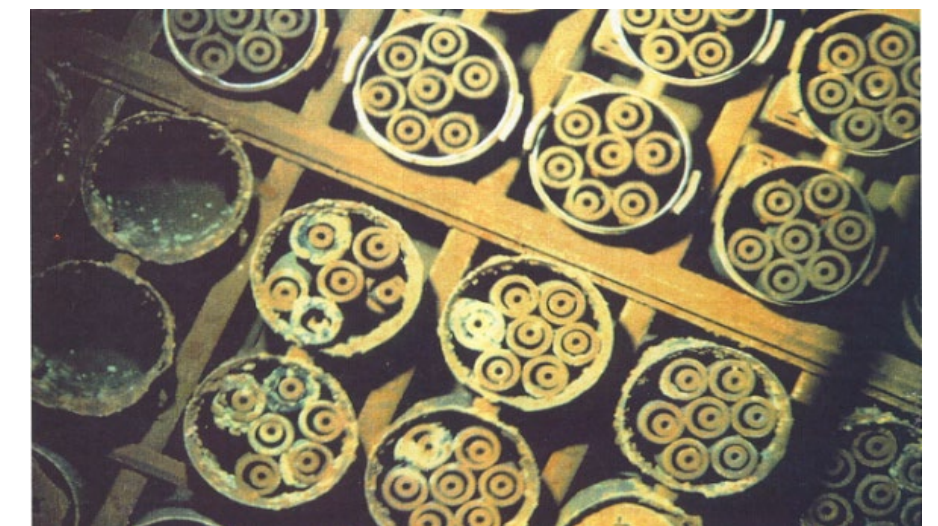
Spent fuel pool at Hanford K Reactor
