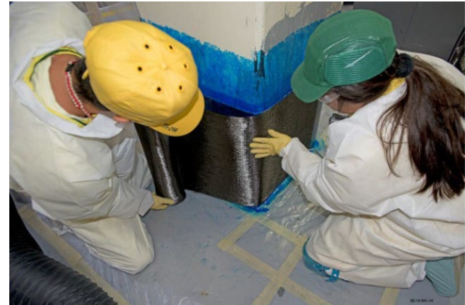
Fiber Wrapping of Structural Columns
