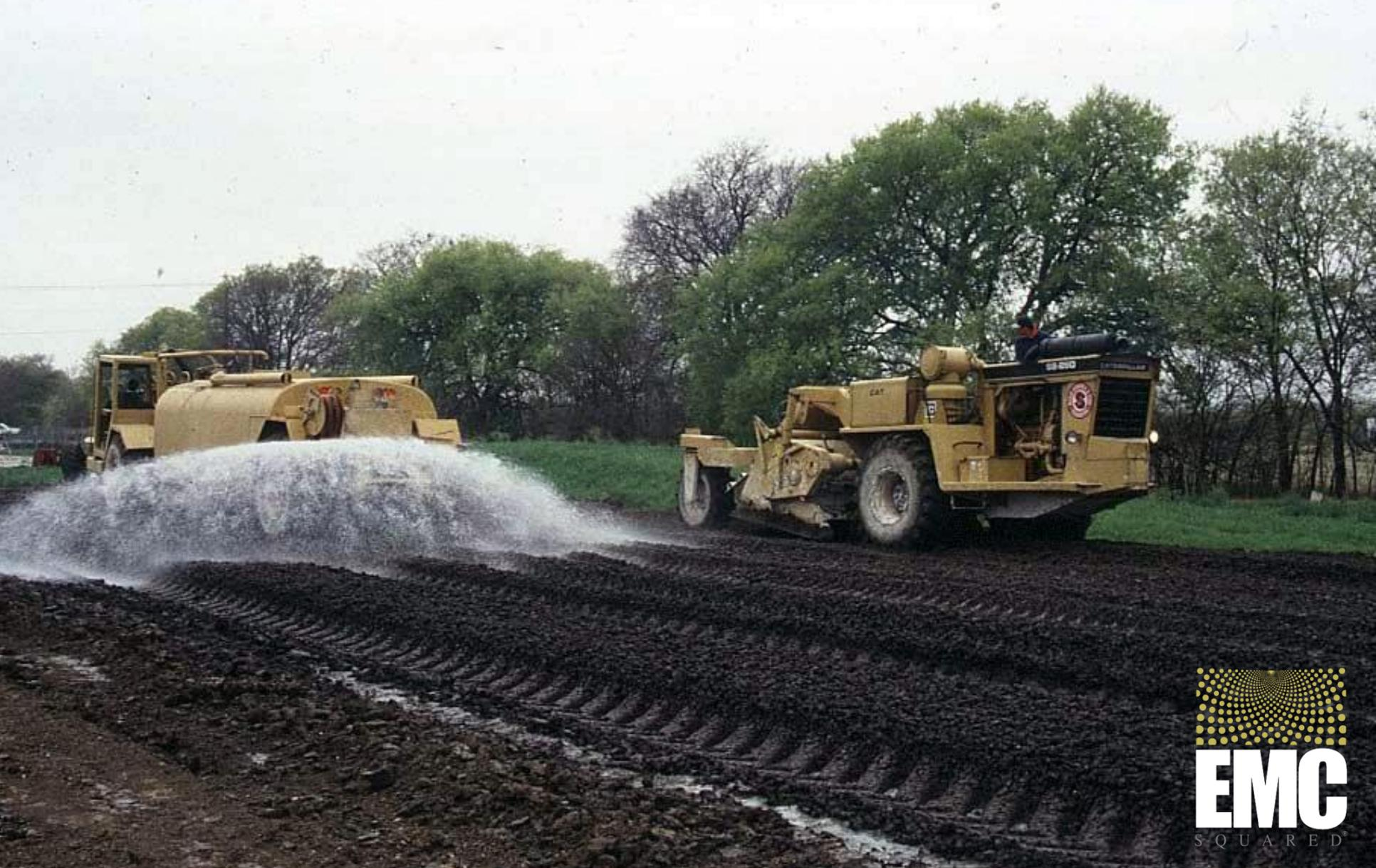
Application of EMC SQUARED<sup>®</sup> System Treatment by Water Truck
