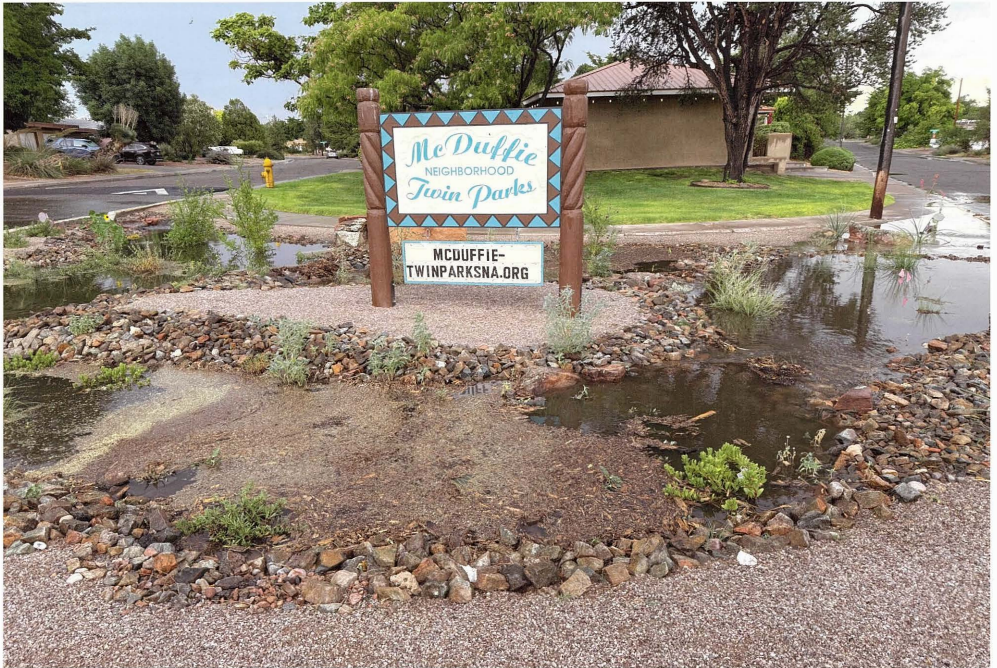
A series of stormwater harvesting basins fill during a large monsoon storm event (July 2026) at the Morningside community-green stormwater infrastructure project in Albuquerque . Image credit: Margaret Keller, community leader.
