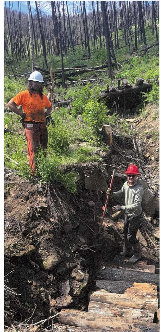
Restoration crew in the Hermit's Peak/ Calf Canyon burn scar, building a log mattress to stabilize a deep gully. Image credit: Reid Whittlesey, Rio Grande Return
