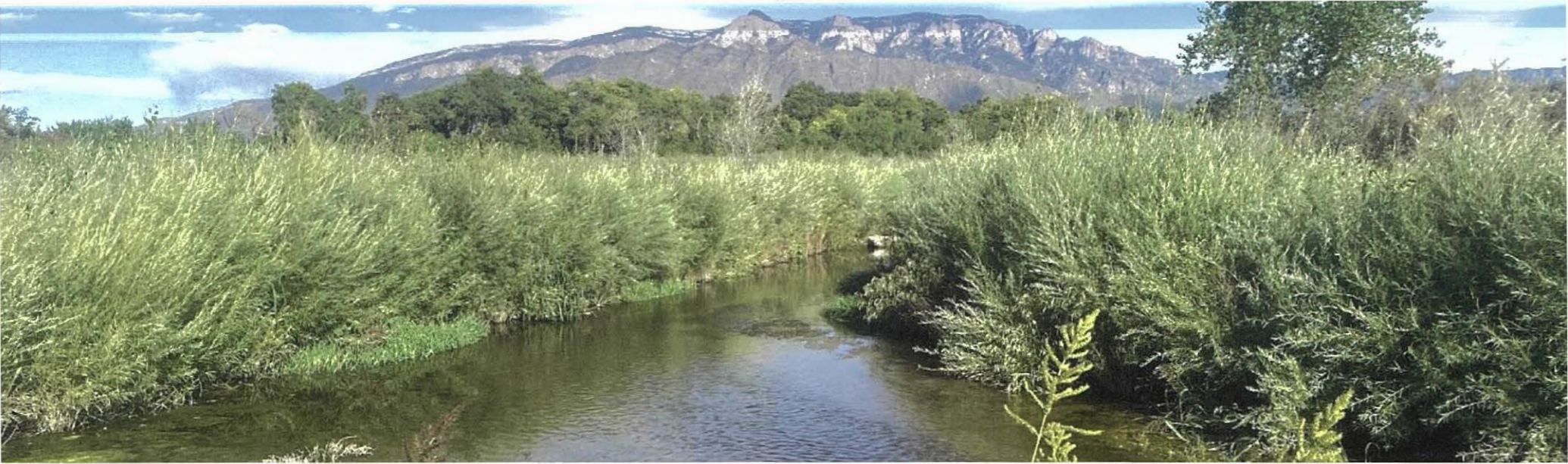
Harvey Jones Bioswale, a green stormwater infrastructure feature that provides wildlife habitat and slows stormwater and treated wastewater before it enters the Rio Grande in Corrales. Image credit: Todd Lopez, Rio Grande Return.
