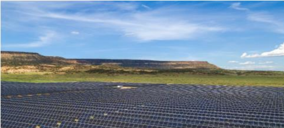
Route 66 Solar Energy Center in Cibola County
