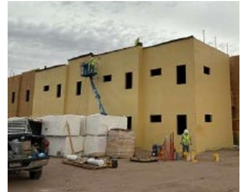
Amador Crossing, Las Cruces. The 50-unit affordable housing development will serve households earning up to 80 percent of area median income. The $15.6 million project includes about $2.0 million in state funding and $4 million in city funding; construction began in February 2025 and is expected to be substantially completed in December 2026.
