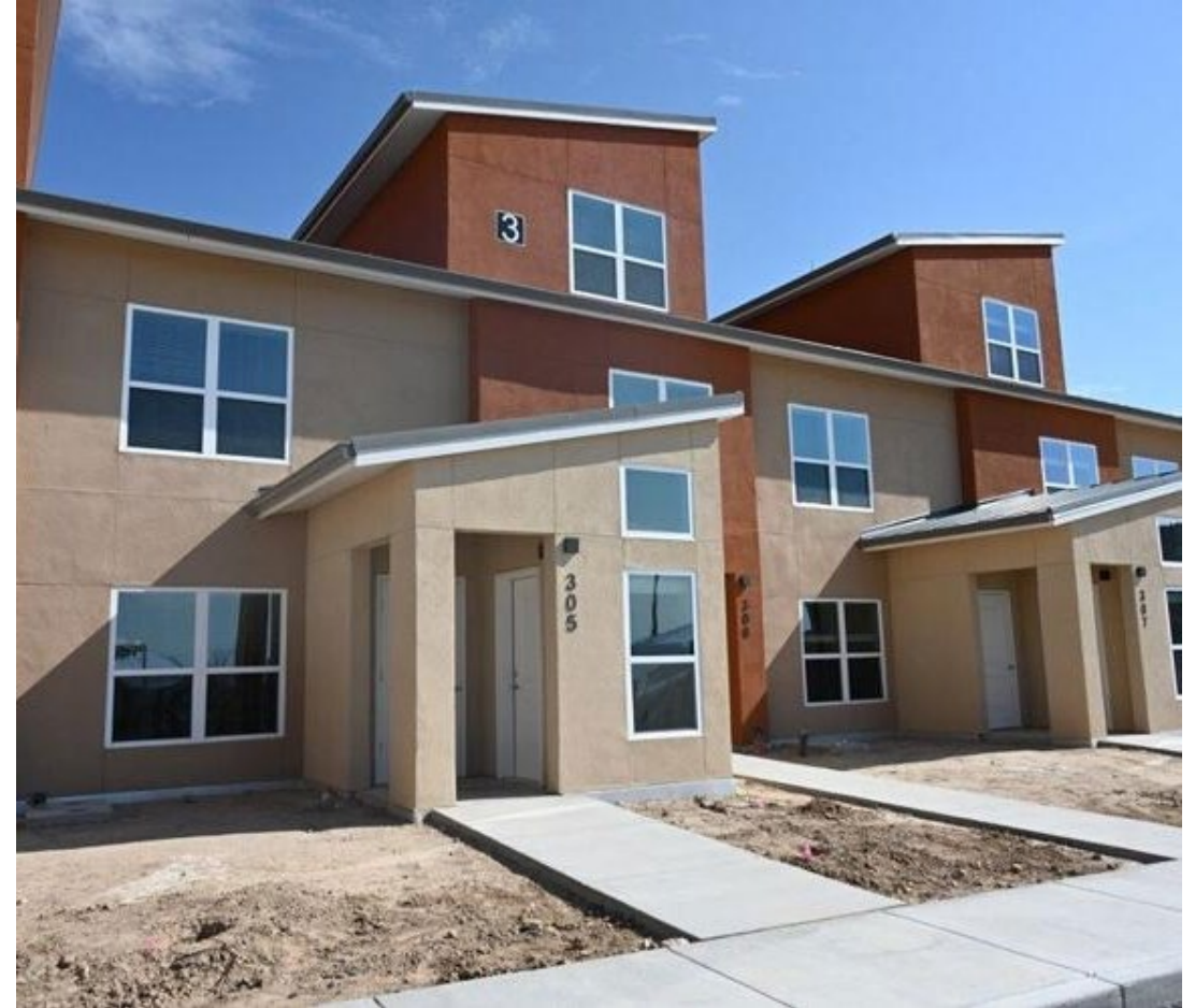
East Paraje Townhomes, a 20-unit development in Laguna Pueblo, New Mexico. Housing New Mexico provided $9.3 million in financing to the project.
