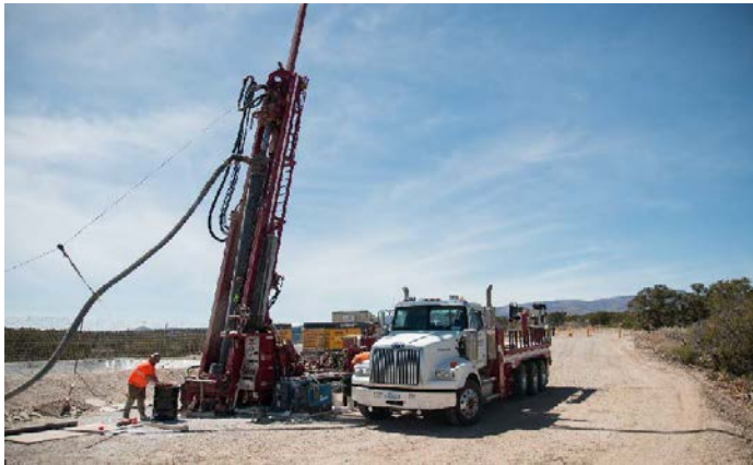
Workers use an angled drilling rig at the CrIN-4 site
