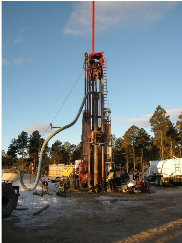
Drilling activities continue year-round at R-68
