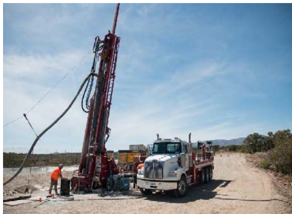
Angled drilling at the injection well CrIN-4
