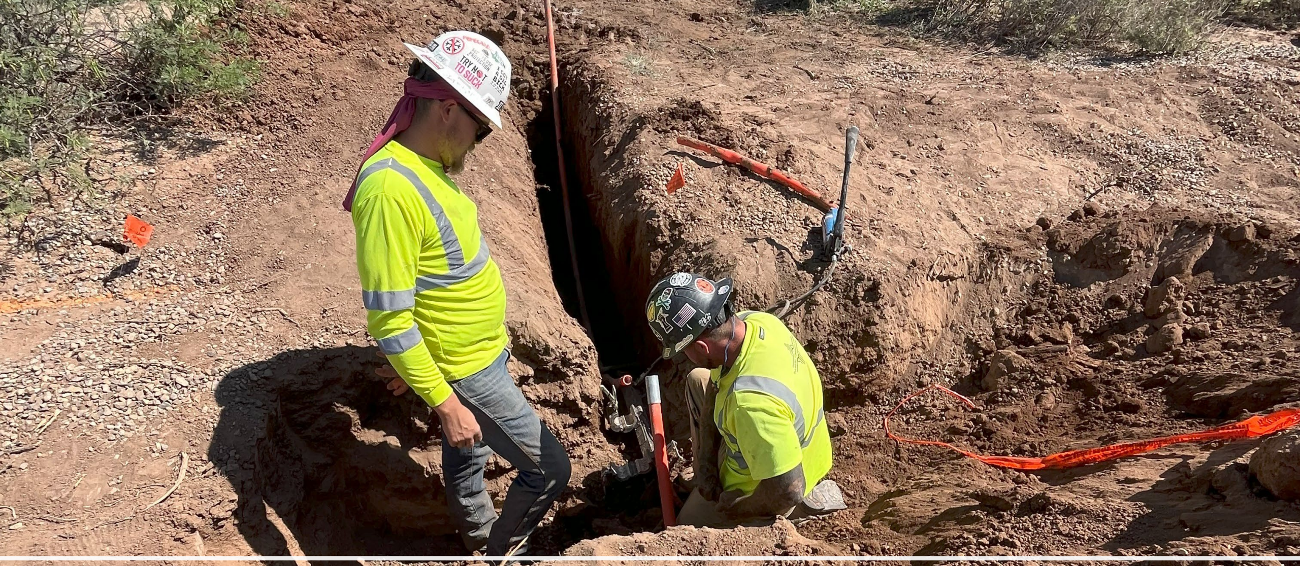
Broadband Project #4 - Trenching (Tularosa Communications – Lincoln/Otero County Project)
