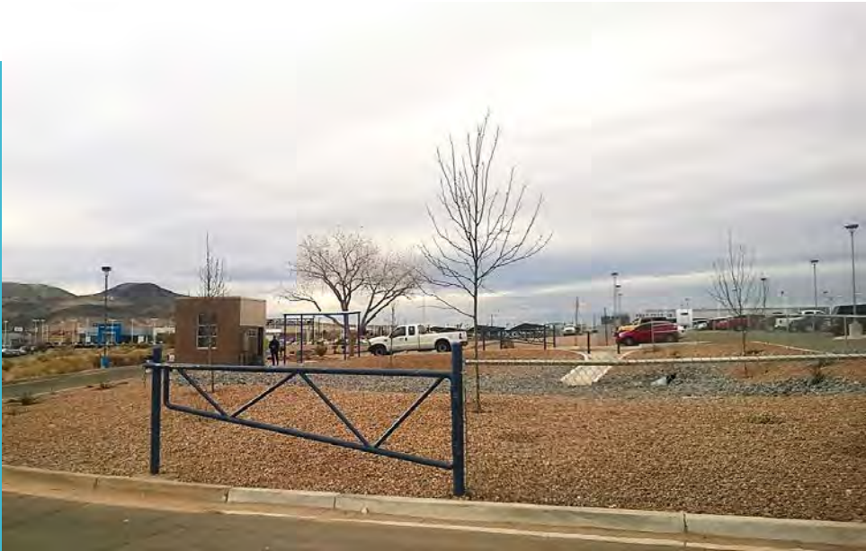
Vehicle Gate and Guard Shack
