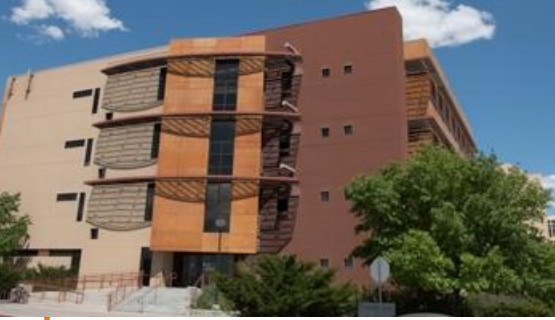
UNM Cancer Research Facility
