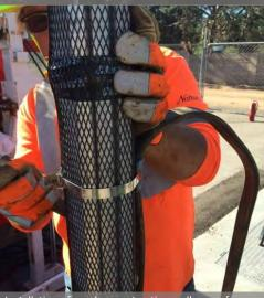
Installation of anode on extraction well pump for corrosion protection (Summer 2016)
